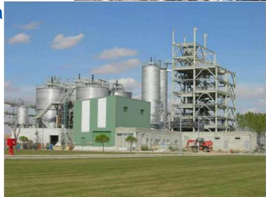
BCyL cellulose ethanol pilot plant ABNT, Salamanca, 5 Million L EtOH / year
